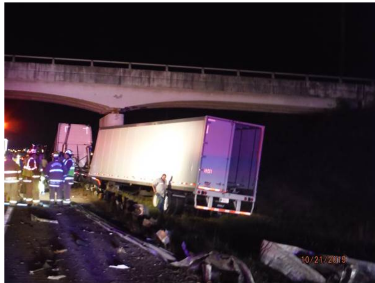
Figure 1: Semi-trailer truck impact on Elrod road bridge
