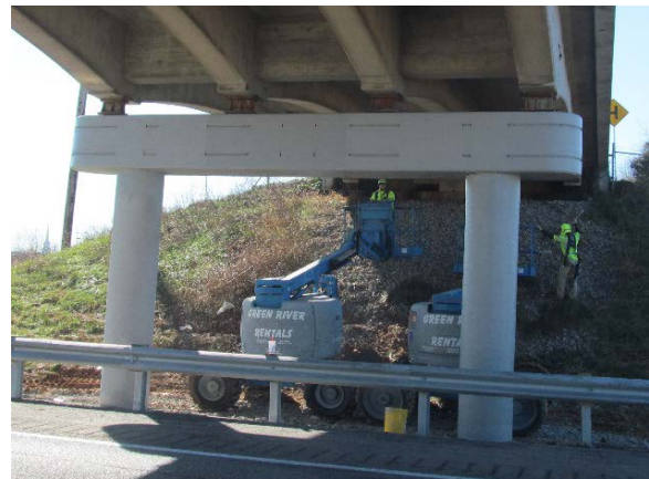
(b) Following application of protective coating
