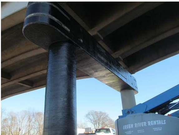
(a) Pier after CFRP wrapping
